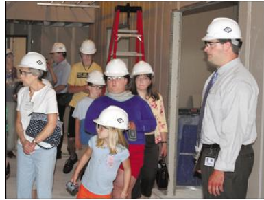
Project Manager Matt Nolan narrates one of several tours of the addition to Elizabethtown Community Hospital. All of the visitors are in OSHA compliance with hard hats and safety glasses. Staff Photo/Alvin Reiner /
